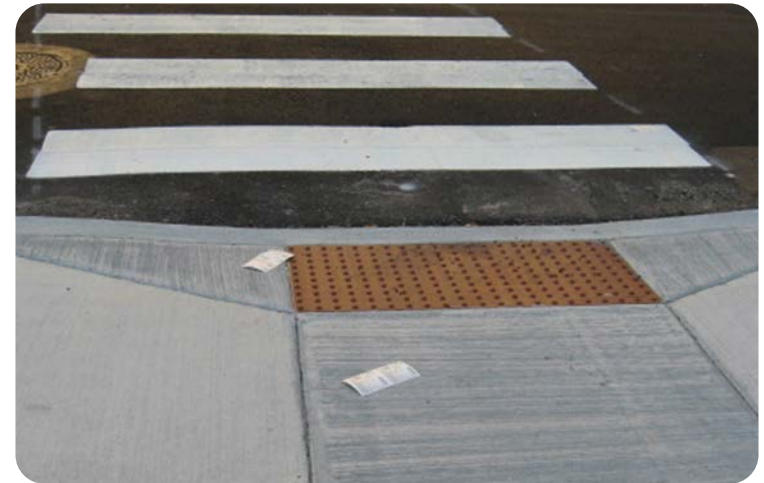
An ADA-accessible curb ramp installed in Dunn.
