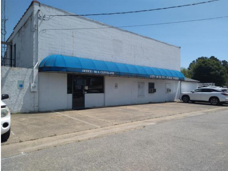
The Public Works parking lot has an ADA accessible parking space; however, it is not van accessible and lacks an access aisle. Parking spaces should be re-striped so that the space closest to the entrance of the building is van accessible and has an adjacent 8-foot wide access aisle. The accessible parking space should also be marked with the International Symbol of Accessibility on the pavement and the fine imposed for parking without the proper permit.
