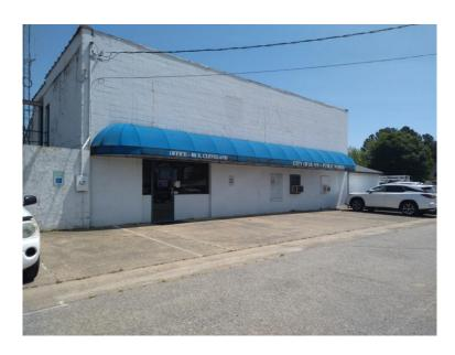
The Public Works parking lot has an ADA accessible parking space; however, it is not van accessible and lacks an access aisle. Parking spaces should be re-striped so that the space closest to the entrance of the building is van accessible and has an adjacent 8-foot wide access aisle. The accessible parking space should also be marked with the International Symbol of Accessibility on the pavement and the fine imposed for parking without the proper permit.
